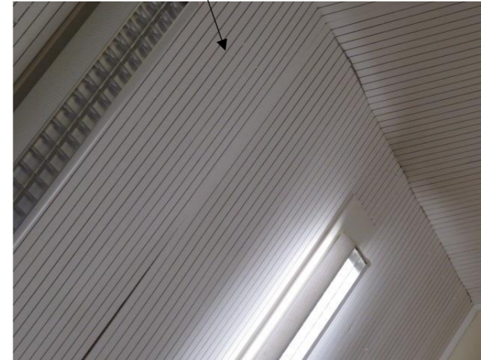
Internal view showing plastic ceiling panels
