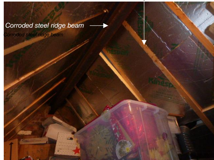
View in roof space
