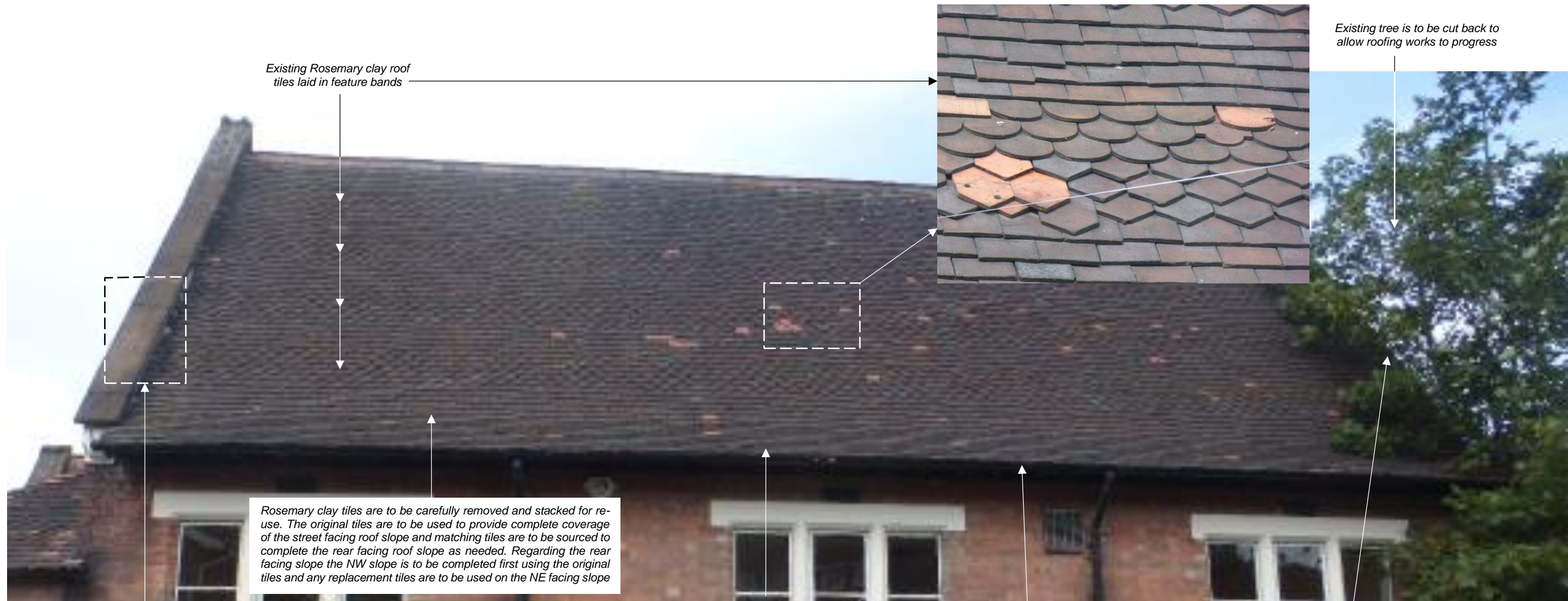
Gutters are to be cleaned out and all support bracket fixings are to be checked and repaired as necessary
