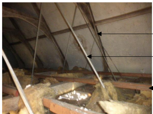
View in roof space showing trusses, ceiling beams and metal ties
