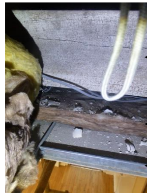
Suspended ceiling grid underneath trusses, with insulation quilt directly over
