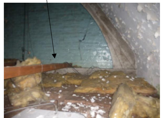
View in roof space showing gable end wall
