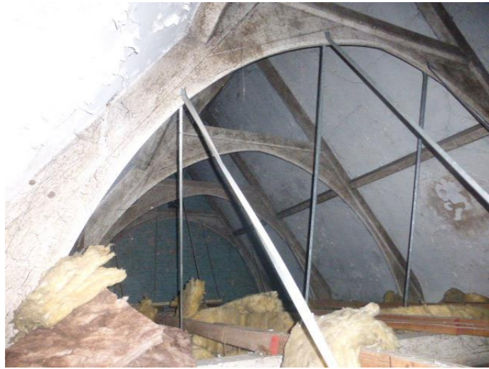
View inside existing roof space
